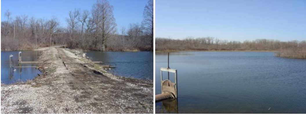
Gated culverts on Fowler Lake
